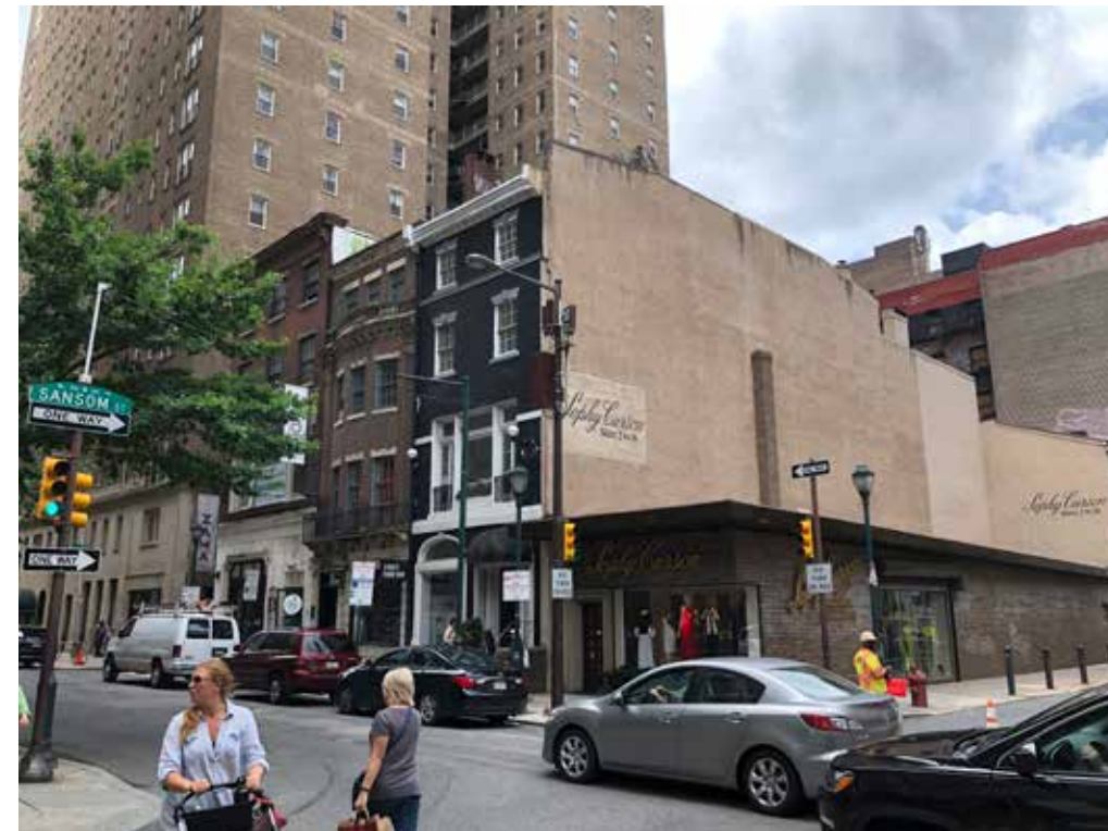
8 Looking Southwest on 19th and Sansom St.
