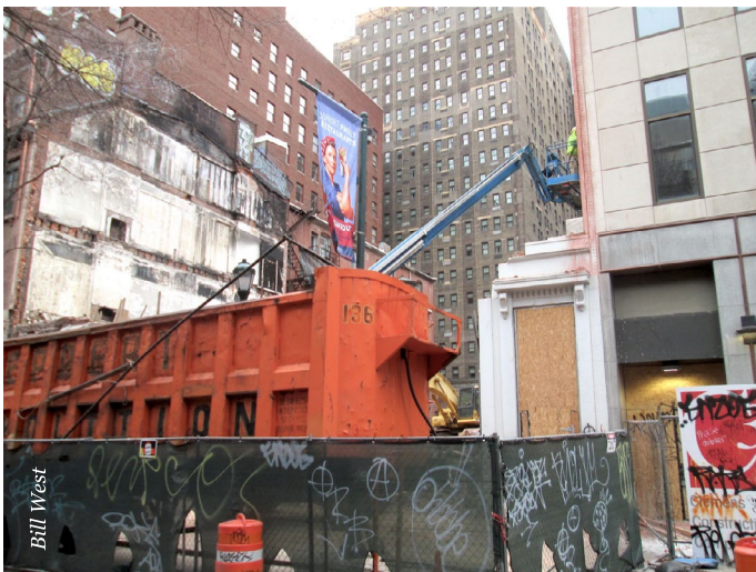
Scene of demolition in progress on the 1700 block of Walnut.
