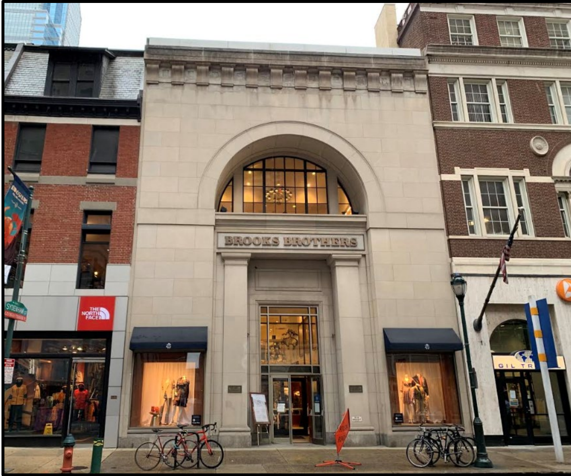
Figure 3. The south elevation of the subject property. Source: Oscar Beisert, 2019.
