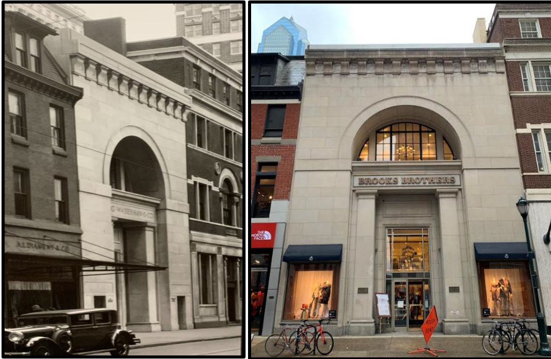
Left: Figure 1a. A view of the subject property just after it was built in October 1930. Source: Walnut Street Files, Penrose Collection – Photographs, the Historical Society of Pennsylvania; and Right: Figure 1b. The south elevation of the subject property. Source: Oscar Beisert, 2019.
